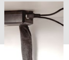
Soft Cable Management
